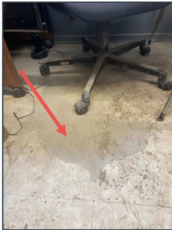
Photograph 4: Fair Condition asbestos-containing 12" x 12" (30cm x 30cm) beige with red streaks vinyl floor tiles in the Public Works Garage Office (Englobe Sample ID: 02A-C).
