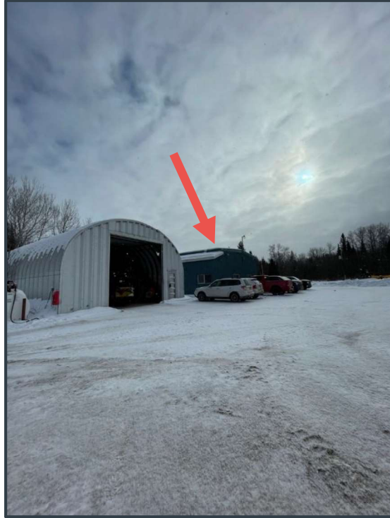
Photograph 1: Public Works Garage
